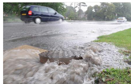
Fig. 2.3 – sewer surcharge
